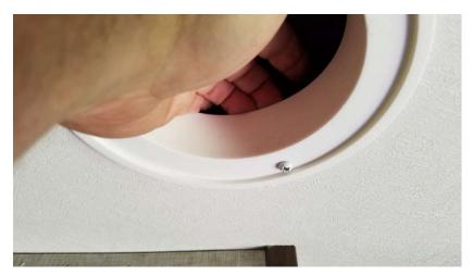
When I removed the vent cover which exposed only the cover housing, it would be easy to miss the problem. But once you feel around as I did in the photo, you will likely find several large gaps between the plastic housing and vent duct. Here I can fit my fingers in the gap. The next photo will show better the problem.
