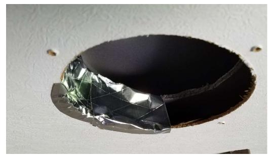
To fix, I used good quality duct tape to seal the void. Note I said DUCT tape, not DUCK tape. This is the good stuff you find in the heating isle. It is a heavy tin foil tape with very sticky adhesive. I found 4" strips worked best, and I overlapped each about 1/2"
