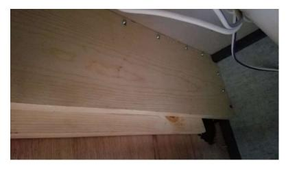
I used two pieces of 1 x 8 to make a support inside the counter to screw the brackets to. Without this, I fear any heavy load on counter extension would cause the thin panel wall to fail.
