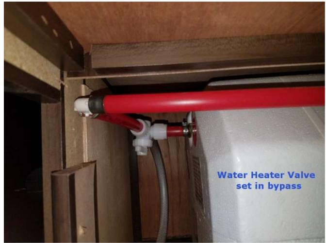
Above shows the hot water tank bypass valve in normal and in bypass mode.
